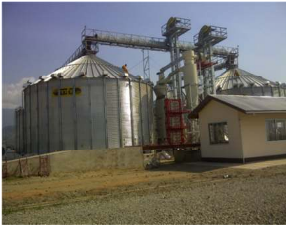
Bucket elevators & belt conveyors
