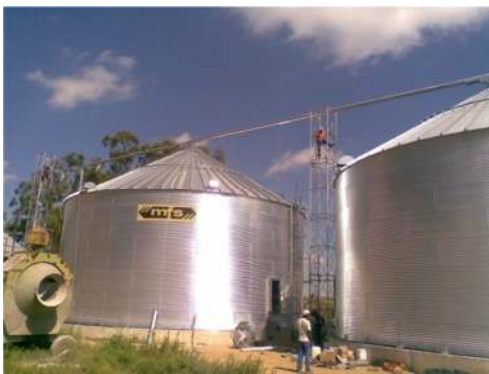
An un-stiffened bin: Farm/drying/ heavy duty bin
